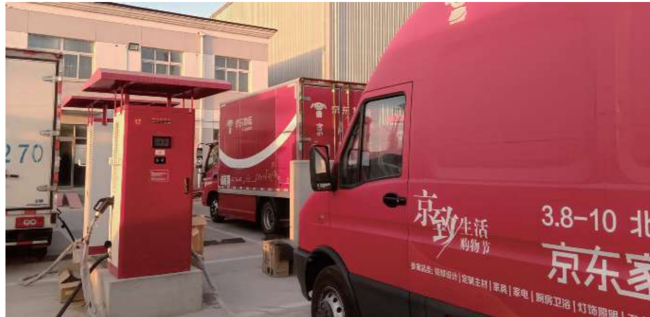
JD (Beijing Majuqiao) Logistics Park Charging Station
